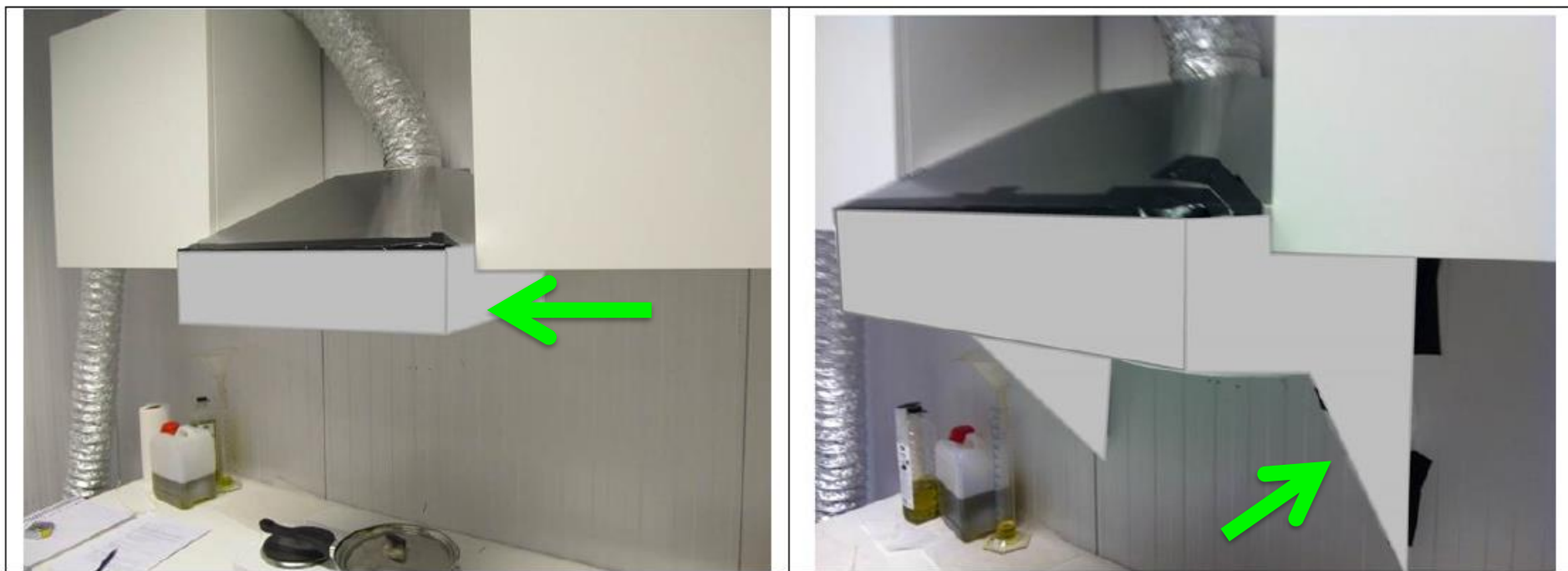
Figure 2. Left: damp buffer applied in experiment G, Right: damp buffer with side barrier in experiment H and I.
