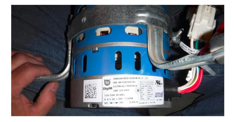
After Improving air flow, we are able to change out the inefficient permanent split capacitor motor (PSC) with a replacement ECM (Constant Torque). The drop in wattage (same airflow) is often very significant.
