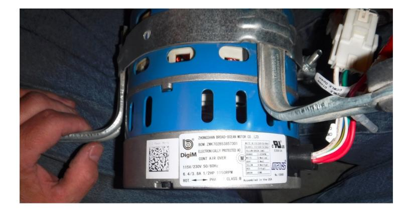
This model also allows us to set up a very low continuous movement of air for filtration, ~400 - 700 CFM, @120 - 180 Watts of power.
