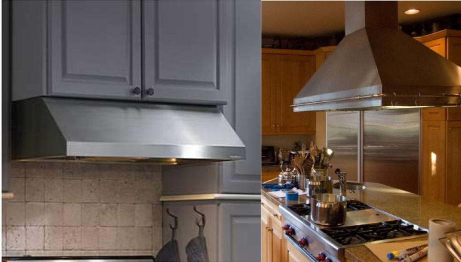
Deep hoods with large internal volumes, and full coverage of cooking surface, are more effective at capturing cooking emissions. Left: Ducted (vented) range hood. Right: Wall installation. Images: B. Singer, LBNL.
